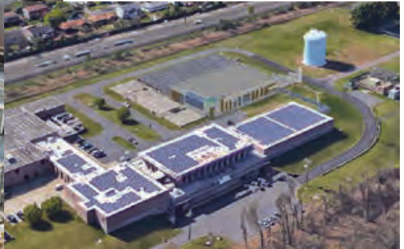
Rendering of the planned upgrade to the Carl J. Olsen Surface Water Treatment Plant
