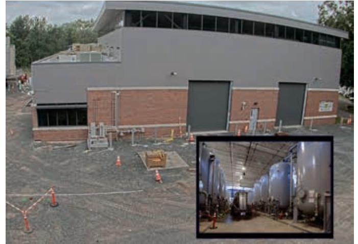
The Park Avenue facility is now complete, in service and treating groundwater for PFAS Compounds. Below are vessels used for granular activated carbon filter treatment.
